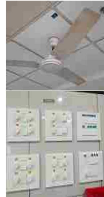
Identification stickers pasted for switches, regulators, fans & light fixtures.
