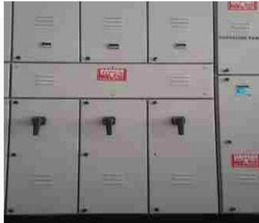
SSB - cleaned and repainted
